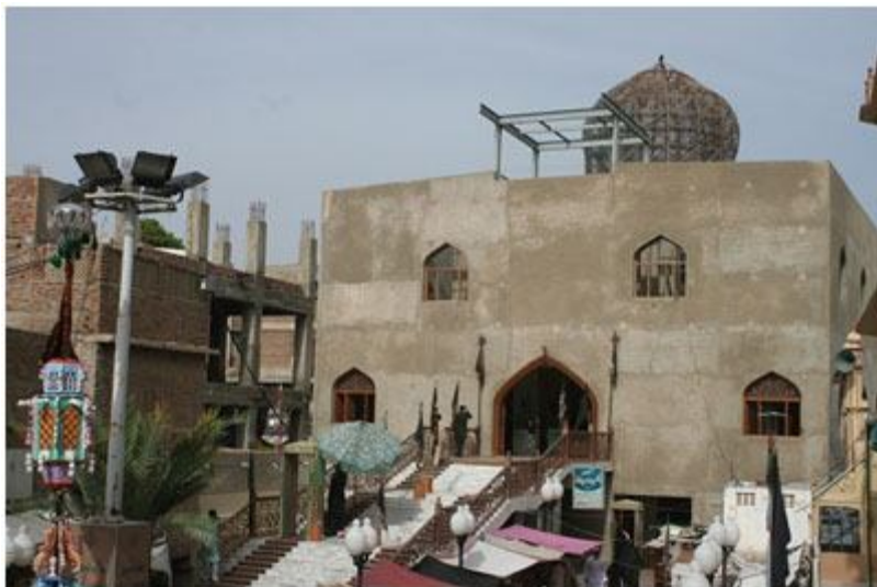
Fig. 5 View of under construction shrine of footprints of Imam Ali at Hyderabad
