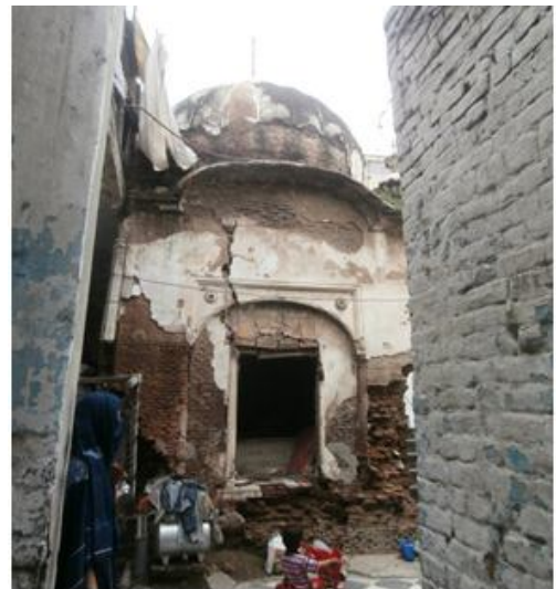
Figure 15. Side view of the Gurudawara.
