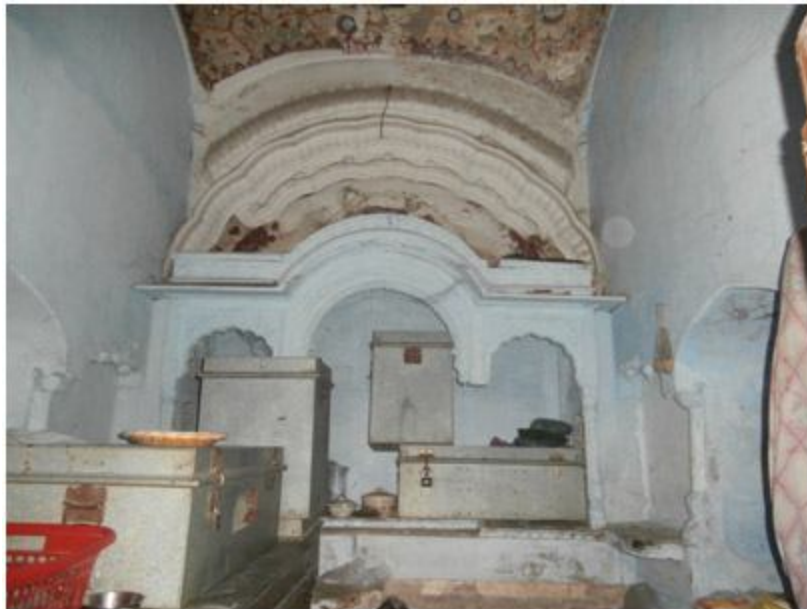
Figure 6. View of the central niche of the garbhagriha.
