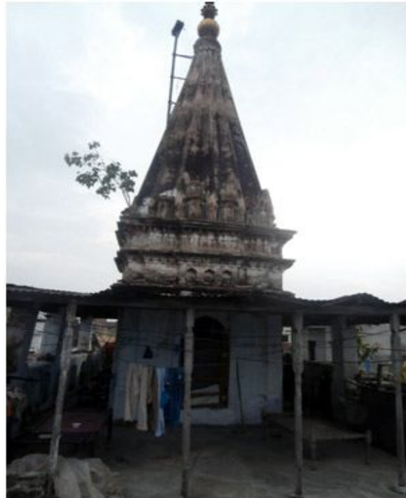
Figure 1. Jain temple, View of Shikhara from the roof.
