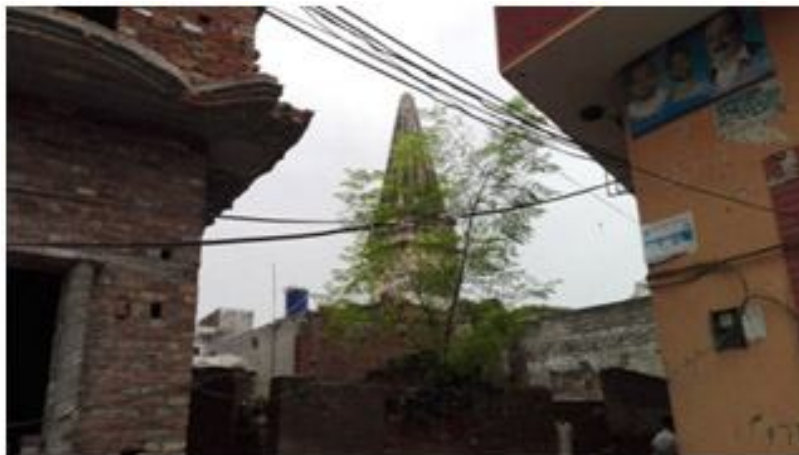
Figure 9. Hindu Temple as seen from outside.
