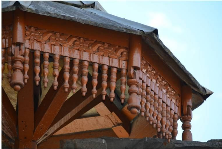
Figure 6: Intricate detailing on the fringes placed at the copula of the temple shrine (Source: Author)
