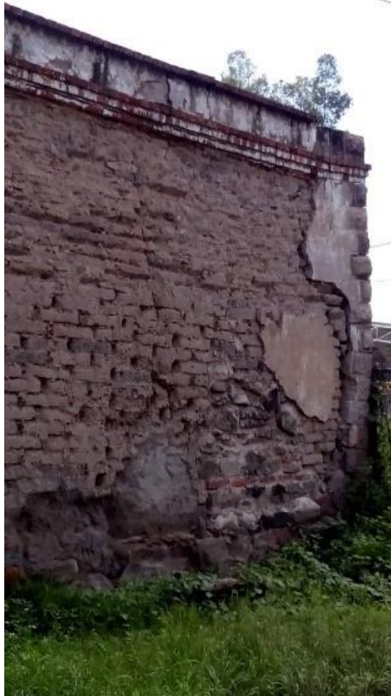
Figure 2. In the federal area, belonging to the National Railways of Mexico ( Ferrocarriles Nacionales de México – FNM), the site shows a vestige of late-19 th -century vernacular dwellings, currently in a fragile state of conservation. Source: the author (2020).
