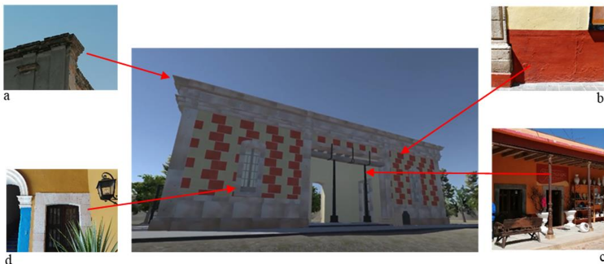
Figure 5. 3D virtual reconstruction of a typical 19 th century railway station (Guerrero Contreras, 2021), with architectural elements that illustrate its morphology. a) cornice, b) wall finish, c) metal column, d) window opening. Museology supported by computer technology results in an inclusive and emotional learning for the audience. Source of photographs a, b, c, d: the author (2020).
